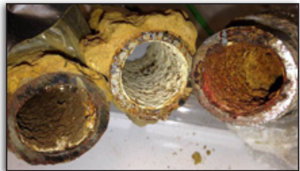
Flint drinking water lead pipes - Google Images
