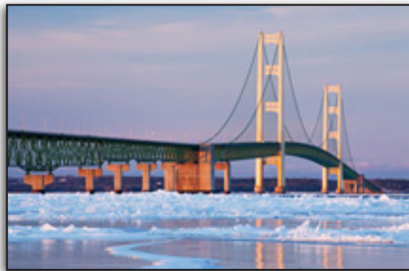
Mackinac Bridge parallels Line 5 pipeline Photo courtesy of www.oilandwaterdontmix.org
